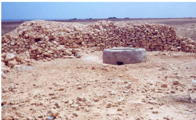
Figure 3.1. Cisterns for rainwater harvesting.
