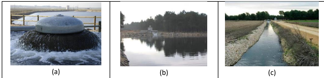
Figures 3.3. Managed artificial aquifer recharge in “El Carracillo” (CEA): (a) control head; (b): settling pond and (c): infiltration channel.
