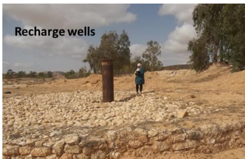
Figure 3.2. One of the recharge wells upstream of the spreading perimeter
