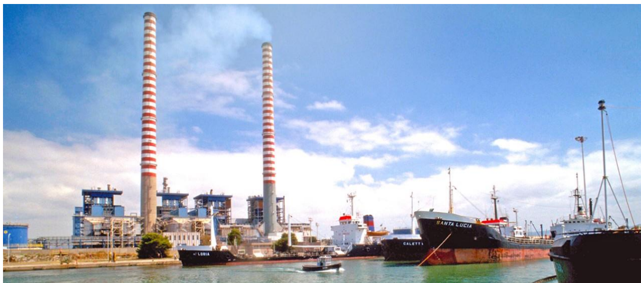
Figure 3.15. The thermal power station in Piombino (source: https://corporate.enel.it/it/futur-e/impianti/piombino ).
