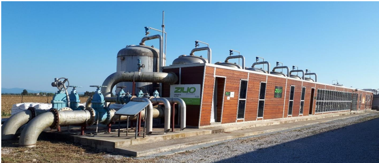
Figure 3.8. Treatment scheme for Boron in groundwater in Franciana (run by ASA spa).
